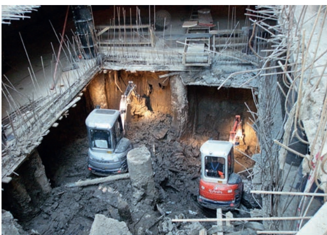
Elite complex of residential and office buildings with a three-storey underground parking. The project using the technology of construction of the underground part of the structure (depth - about 11 m) according to the top-down principle. St. Petersburg, Zoologicheskoy per., 2-4
