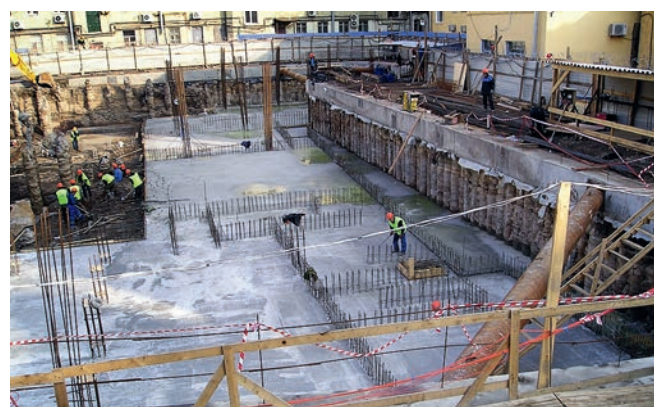
Boris Eifman Dance Academy. The design of the enclosing structures of the pit (depth - 6.3 m) from tangential piles, the pile foundation from bored piles, united by a monolithic reinforced concrete grillage of variable cross-section, reinforced concrete structures of the ground floor. St. Petersburg, Liza Chaikina st., 2
