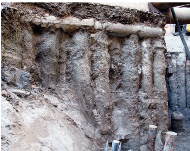
Reconstruction and restoration of the Eastern Wing of the General Staff of the State Hermitage Museum. Project for the adaptation of basements (depth - about 5 m) for museum purposes, replanting foundations for load-bearing walls on root piles in conditions of limited space and watering of the foundation soils.
