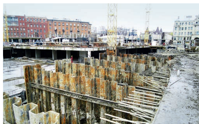
Residential complex Lumiere with built-in and attached premises and a two-level underground parking lot. Design of the enclosing structure of the pit (depth - 6.6 m). St. Petersburg, Korpusnaya st., 9
