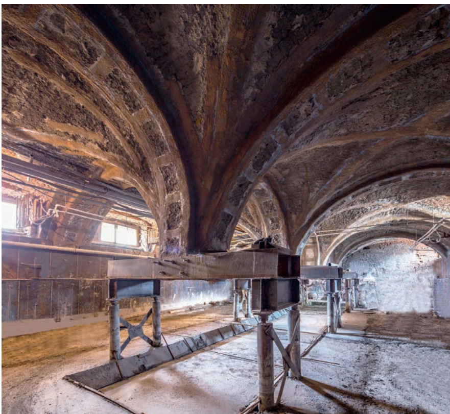
Alexander Palace. The Tsarskoye Selo State Museum and Heritage site. Reconstruction, adaptation for modern use. Hanging of historical columns on the GEOIZOL-MP root piles with the addition of new foundations. St. Petersburg, Pushkin.
